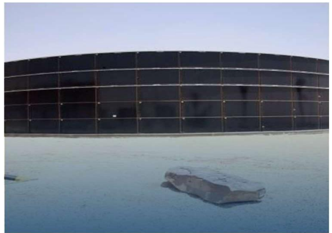
Steel water tanks
